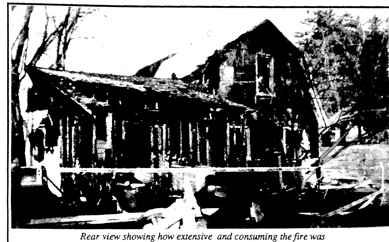
Rear view showing how extensive and consuming the fire was
