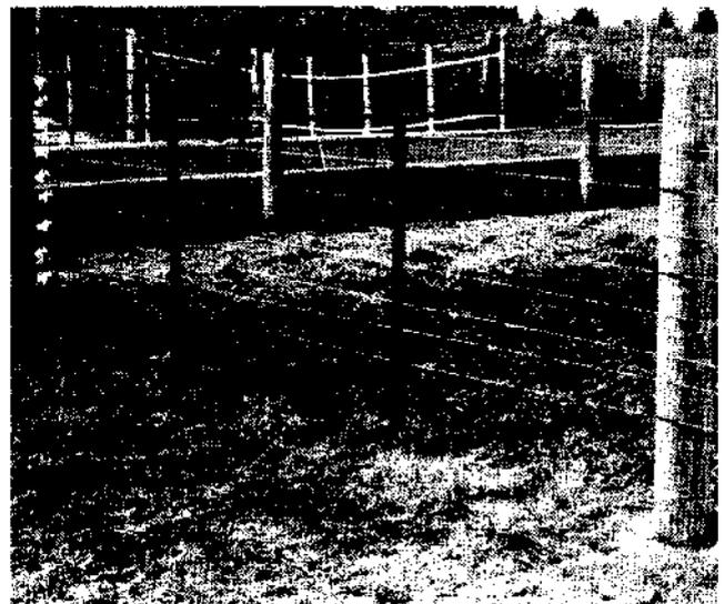
Figure 1. This photo shows many of the components of an electrified high-tensile, smooth wire fence for a feedlot or a cow drylot: 9 wires with the 1st, 5th and 7th electrified (note wrap-around plastic insulators); 2 posts, 32-ft. spacing; 2 wooden droppers; 9 in-line strainers to tighten fence.
