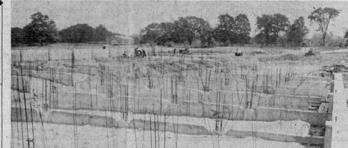
SHOWN in this picture are the foundations for 25 storage and curing bins at the Kalamazoo fertilizer plant now under construction. Each bin will hold about 600 tons of material. The steel rods were to be bent at right angles to reinforce the concrete floors to be laid. Structural steel pillars for the roof and sides of the bins will rise from the depressions in the footings. Sides of the bins will be wood. Materials will be brought to the bins by overhead belts. Removal of plant food and raw material from bins will be done with power shovels that scoop up a ton.
