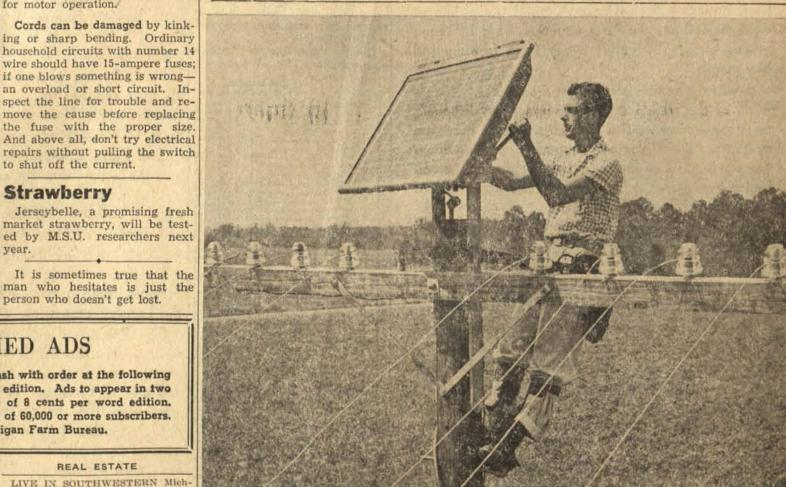
The Bell Telephone Laboratories Solar Battery being mounted on a rural telephone line near Americus, Ga.
