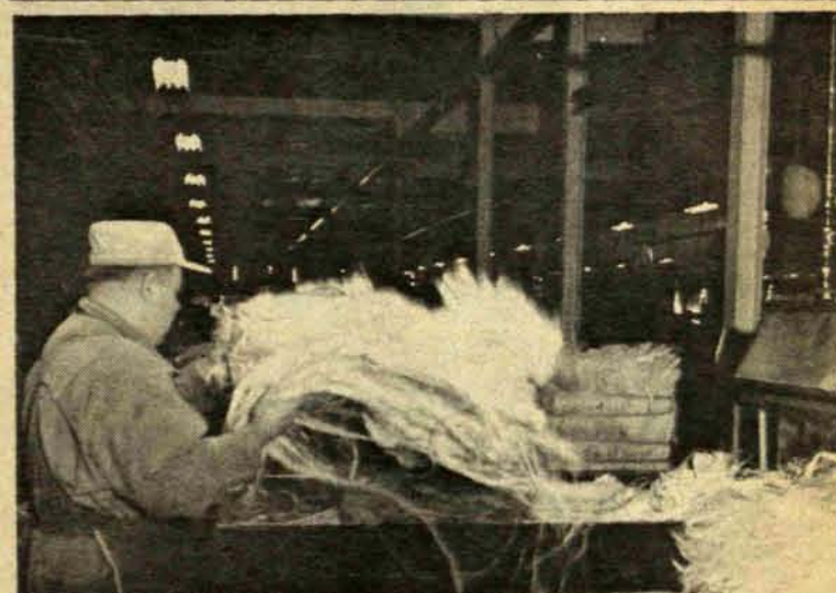
HARD HANDWORK—controls the flow of "sliver" into the first in a row of eight combing machines at the Brantford, Ontario, Cordage Company. Here the raw fiber is tossed onto a tray-like belt containing hundreds of spiked "combs."
