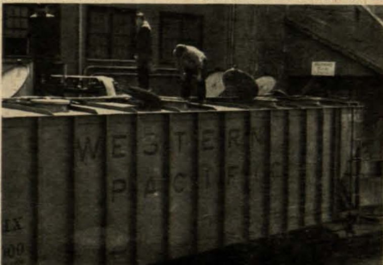
LARGER CARS, — LOWER COSTS. Farmers gain by use of new giant, stainless steel freight cars, designed especially for bulk shipments. Grain and beans move quickly into the car through any of 12 loading ports, or out through discharge gates at the bottom of each compartment.
