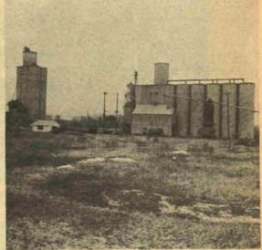
STORAGE COMPLEX — east of Charlotte, holds grain beans for the Eaton Co-op. Steam pours from the 1,000 bushel per-hour grain dryer. A cluster of "unit-poured" concrete silos for bean storage is part of the complex.
