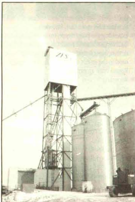
The receiving portion of the ZFS processing facility, including the 165-foot tower; a 1,000-bushel dump pit, capable of handling 10,000 bushels per hour; wet tanks; and the first of four 500,000-bushel storage bins, is complete.
