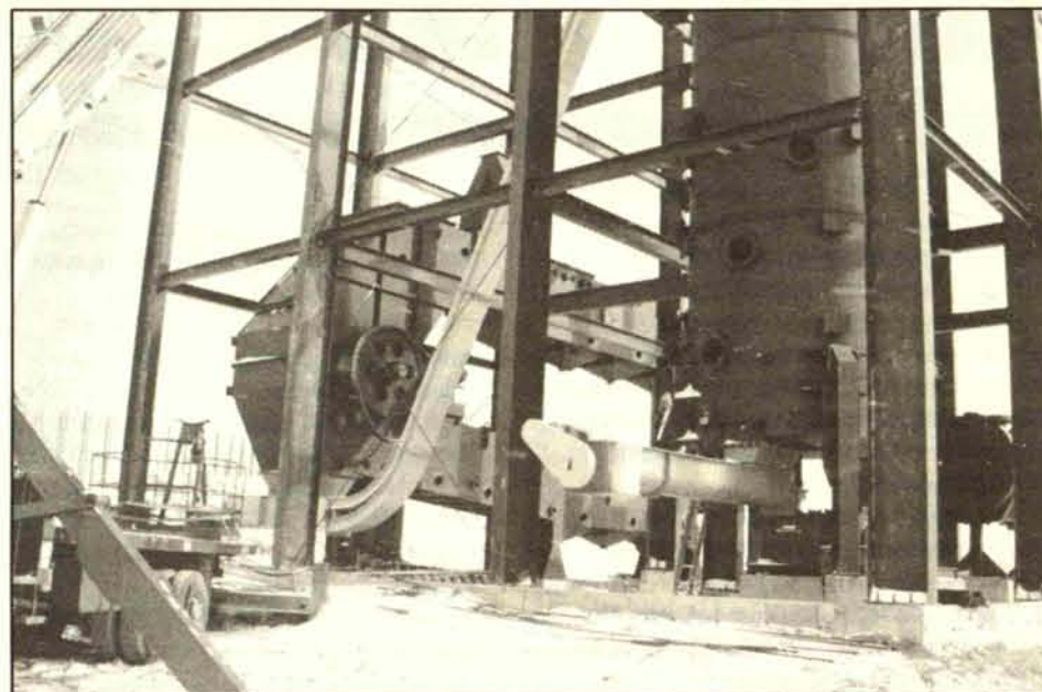
An up-close look at the 150,000-pound extractor where the actual oil is removed from the soy flake. Once the flakes leave the extractor, they enter the top of the structure on the right side, known as the DTDC tower (desolvitizing, toasting, drying and cooling), before the soy flake is sent back to the preparation building for further processing into finished soymeal.
