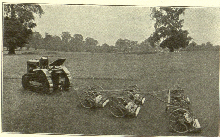
RANSOMES "QUINTUPLE," DRAWN BY A CLETRAC TRACTOR. IT CAN ALSO BE FITTED WITH A POLE FOR A PAIR OF HORSES
