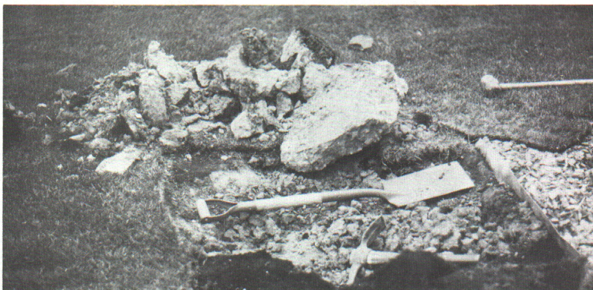
Problems arise when buried debris is not removed prior to establishment.
