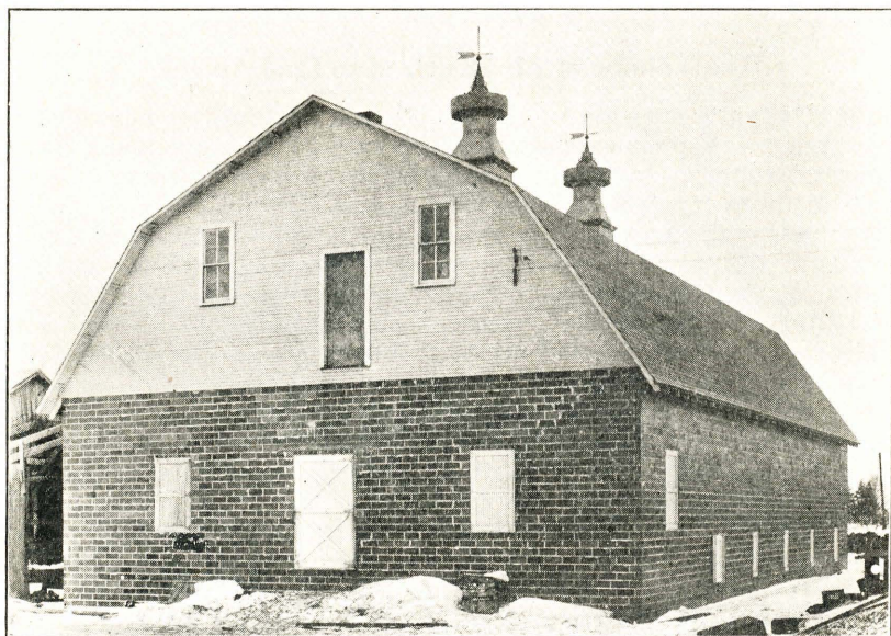
Fig. 23.—Storage K. See Table 2 for description. A double wall of vitrified tile, such as exists here is unnecessarily expensive.
