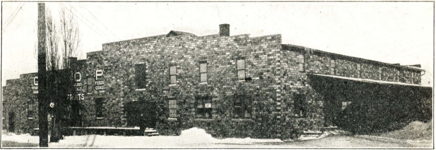
Fig. 25.—Storage O. See Table 2 for description. The apple storage is in the basement of the right half of this building. The basement of the left half constitutes an air-cooled potato storage. The cold air intakes are just above the ground line and most of them are under the loading platforms. A portion of the roof of one ventilator can be seen near the chimney.
