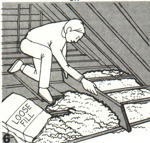
Pour in loose fill insulation between the joists up to the top of the joists. Use a board or garden rake to level it. Fill all the nooks and crannies but don't cover recessed light fixtures or exhaust fans.
