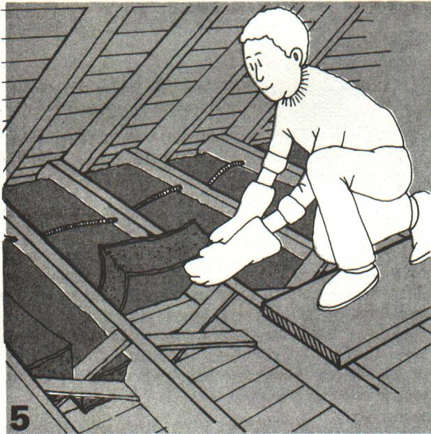
Lay in blankets or batts between joists or trusses. (Note: batts and blankets are slightly wider than joist spacing so they'll fit snugly). If blankets are used, cut long runs first to conserve material, using leftovers for shorter spaces. Slide insulation under wiring wherever possible.
