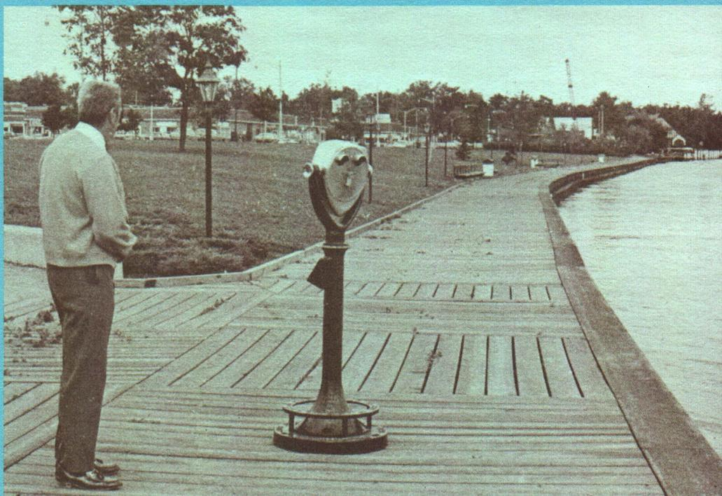
Fig. 14. Board walks of salt-treated wood are worthwhile additions to waterfront parks.
