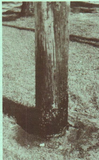
**Fig. 8.** Bleeding poles like this result in preservative loss from upper parts but service life is probably not decreased if not moved. If used as a spring pile some surface oil on water could result.
