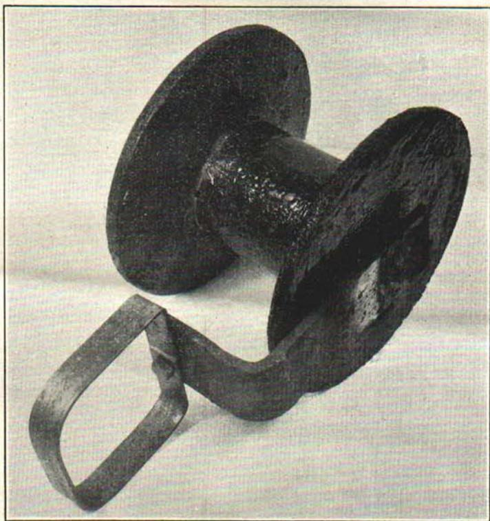
Fig. 10.—The roller used in moving the hose.
