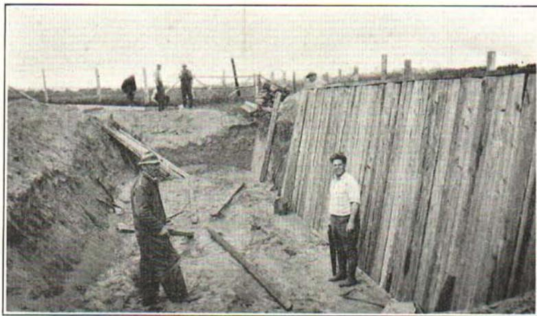
Fig. 4. A trench silo under construction in the Upper Peninsula. Cedar posts were used to line the inside.
