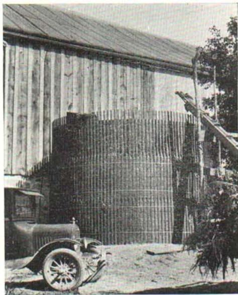
Fig. 1. A well built crib silo, showing details of construction. (Courtesy of American Lumberman.)
