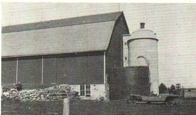
Fig. 2. A temporary crib silo beside a permanent silo.
