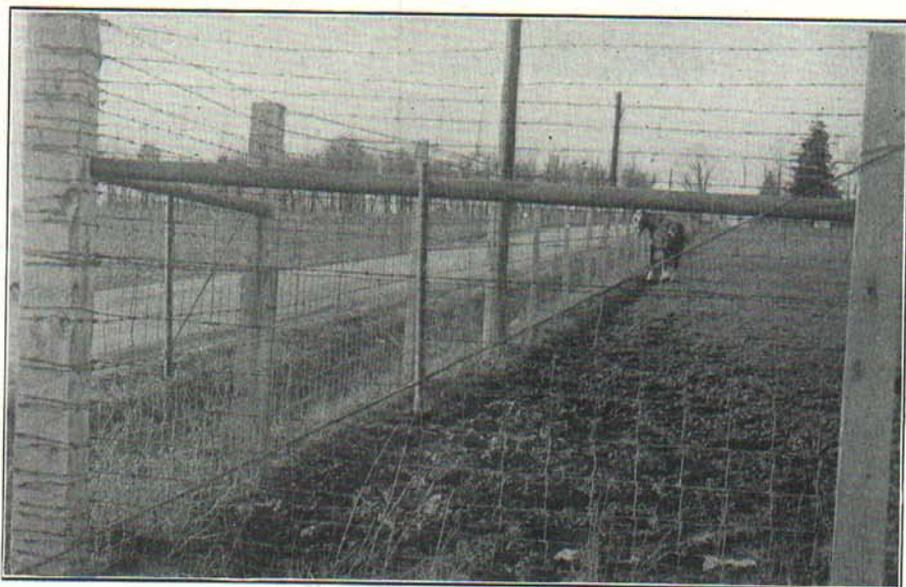
Fig. 8. Wire fencing for stallions. Double-run fence.
