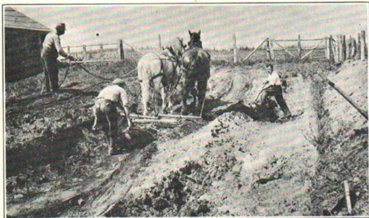
Fig. 1. Excavating for trench silo.
