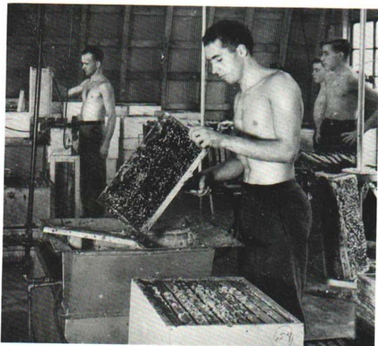
Fig. 27. Uncapping into the cappings melter. In the foreground an uncapping plane, in the background a power uncapper. Note two "merry-go-round" comb tables within easy reach of uncappers.
