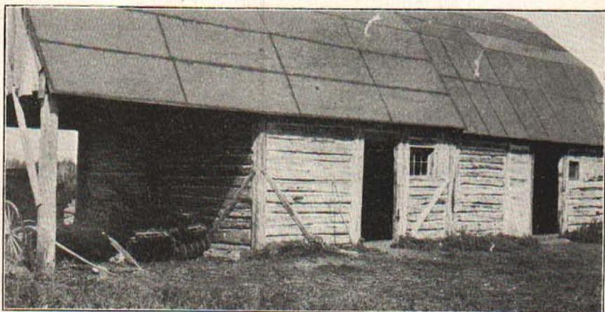
Fig. 19.—Barn made of cedar logs laid horizontally. It would have been better if more windows had been provided. The ends are toenailed to corner logs, instead of the method of notching and crossing used in other log buildings.
