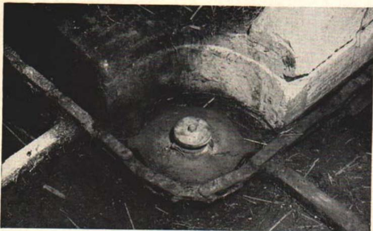
Fig. 20. Corner idler. Note chain construction and steel rail in bottom of gutter which takes all wear.
