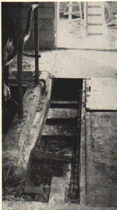
Fig. 17. Part of metal cover removed to show details of slats turning on themselves.
