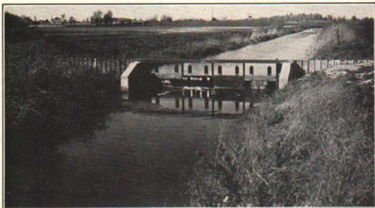
Fig. 1. Dam constructed to maintain water level in a large muck area. Note the use of interlocking sheet steel piling, which is driven deep to extend well out into the bank on each side. It is also driven across the ditch below the bottom of the gates. Concrete piers, concrete apron in the bottom of the ditch, angle iron braces welded into position, and four redwood gates complete the construction.
