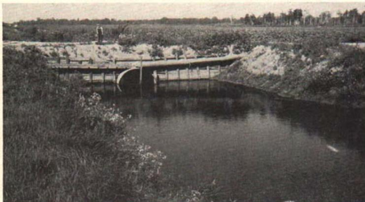
Fig. 4. View of secondary dam and bridge in the Chandlers Marsh drain, nine-tenths of a mile above the master dam shown in Fig. 3. This photograph was taken from the upper side, in late summer, before the retaining planks had been removed to lower the water level.
