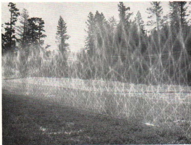
Fig. 5. Perforated pipe lateral in operation.
