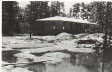
Fig. 8 — Septic tank disposal fields will fail and basements may be wet on soils with mottled or gray subsoil and slow permeability.
