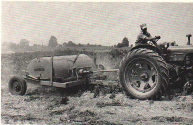
Fig. 8. After the vines have been chemically killed or frosted, the vine beater makes a clean job of the remains for the digger or harvester.
