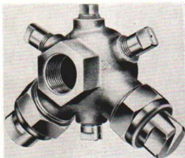
Fig. 18. - Nozzle cluster or "boomless nozzles."
