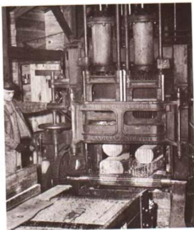
Fig. 17. Sash gang saw measuring 32 inches between styles or sash, with a stroke of 13 inches, depth of cut of 14 inches, and with 15½-inch maximum opening between feed rolls and press rolls. Note individual pressure cylinders actuating the split press rolls to permit feeding of multiple cants. By feeding cants in multiples, the gang-saw can maintain a production of 40,000 board-feet per 8-hour shift. (Photo: Wickes Brothers Division, The Wickes Corp.)
