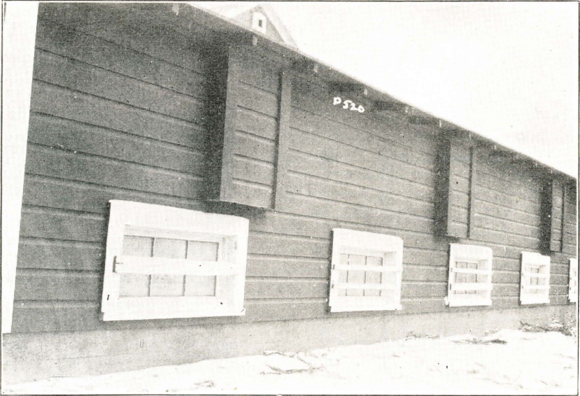
Fig. 9.—Rear Elevation—note the rear windows and the construction of the intake flues.
