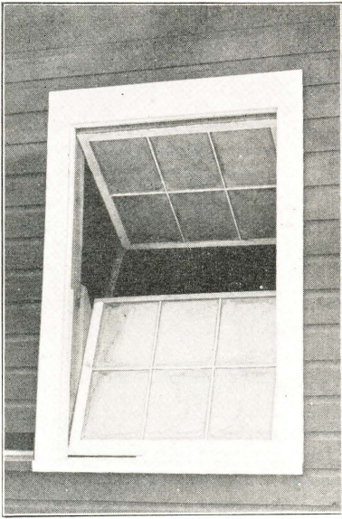
Fig. 4.—Windows arranged to admit direct sunlight—they should be wide open on fine days. The lower sash may be removed.
