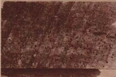
When adult Powder Post beetles emerge, some species leave small holes (shot holes) about the size of a pin in the surface of the wood; others make holes the size of pencil lead. Note the tunneling is to both wood and bark, but primary concern is the damage to the wood.
