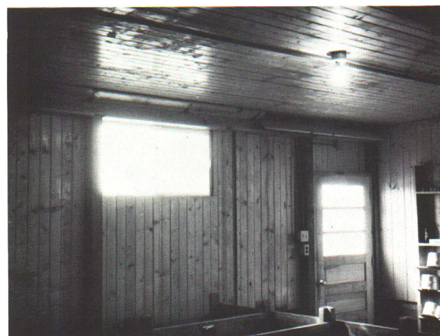
Figure 11 — A 3-inch slot along the ceiling provides space through which dry, cold, fresh air can enter the building. Hinged flaps can be used to deflect the air across the ceiling.
