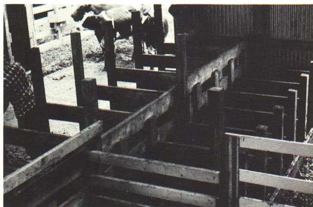
Figure 14 — Different sizes of free stalls should be provided so animals can be moved to larger stalls as they grow.
