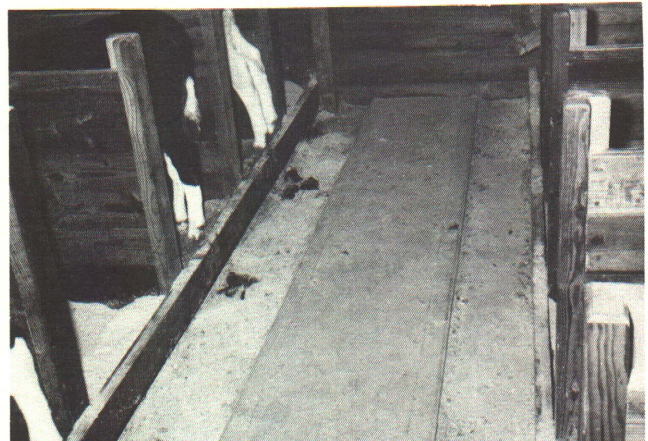
Figure 4 — A shallow gutter behind the stalls collects manure and prevents liquids from running into the alley.
