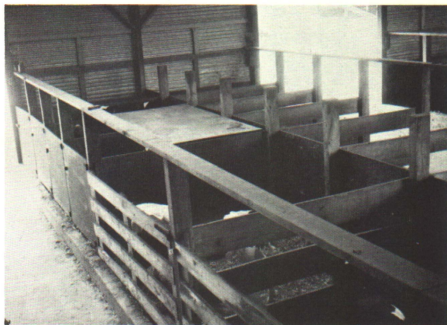
Figure 1—In cold calf housing, a loose pen should have at least three solid sides to prevent drafts. For newborn calves, a plywood sheet over the top forms a cubicle so heat from the calves cannot escape.
