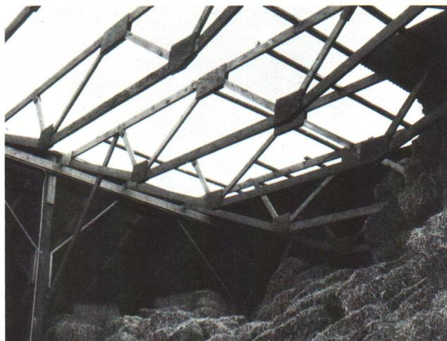
**Figure 11 – Poor nailing of roof girts to trusses caused this section of roof to blow off during high wind.**
