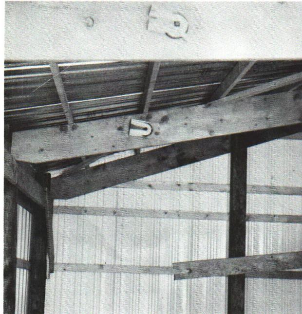
Figure 2 — One-2½ in. split ring was used on this joint where at least two rings should have been used.
