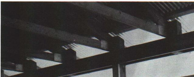
Figure 8 — Truss to rafter-plate joint made with a short 6 in. by 6 in. block.
