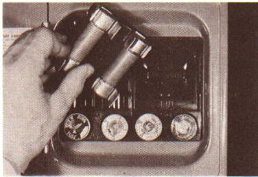
Another type of fuse you will see in the fuse box is the cartridge fuse. These protect appliances which use the most electricity, such as the range, clothes dryer, or water heater. Be sure they are also replaced with the same amperage fuse. Always keep an extra supply on hand of each type and size of fuse you use to avoid inconvenience or problems when stores are closed.
