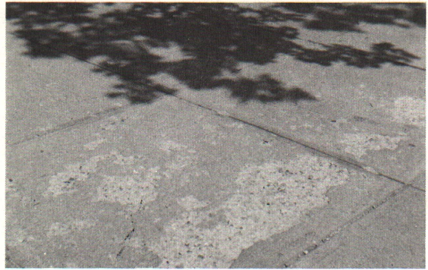
Fig. 20. Too much trowelling to obtain the finish can weaken the surface and cause flaking or spalling.
