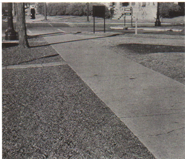
Fig. 32. Crushed brick combines color and utility in this heavily travelled area between walk and curb.
