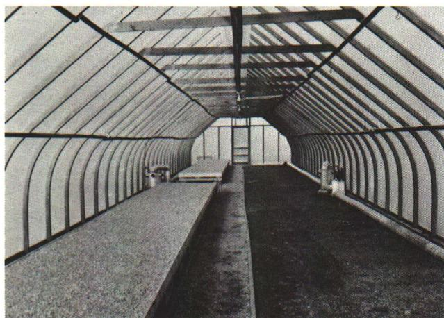
Fig. 8 Interior view of a laminated rafter greenhouse.
