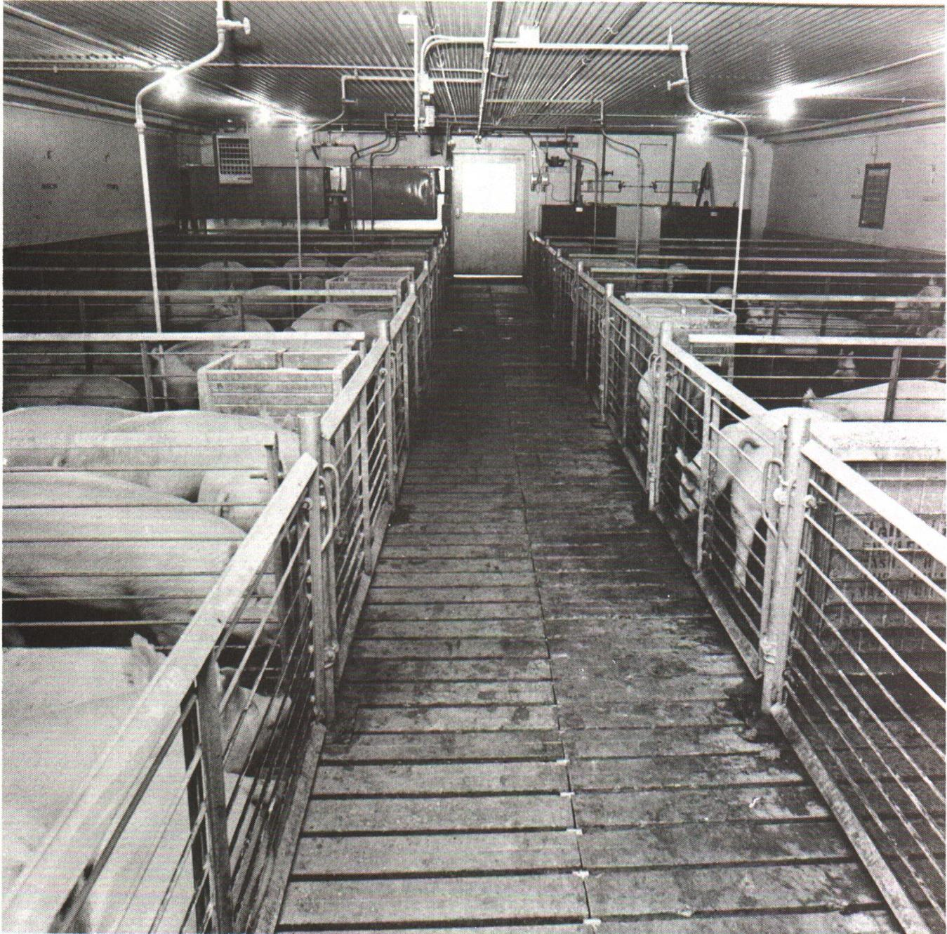
TWO TYPES OF FLUSH TANKS are shown in this growing-finishing facility. The two tanks on the left were made in the MSU blacksmith shop. They dump automatically without any mechanical devices. The tanks on the right are manufactured commercially. The water is released through a door in the front that is opened by a hydraulic cylinder operated off a compressor.
