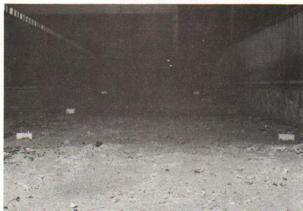
Fig. 5. Stakes in place to give a 2% slope to the floor of the trench.
