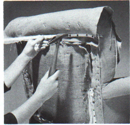
Fig. 53—Blind tacking outside back at top.
