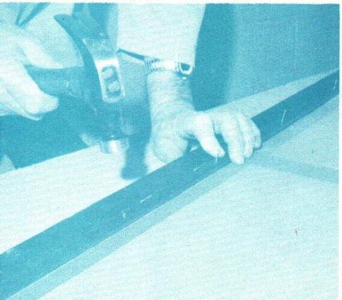
Step 9. Replace the wooden strips around each panel. If they were broken when removed you may have to buy new ones. Paint the entire screen. Keep screen frames painted. When the paint peels off moisture gets into the wood. This can cause the frame to swell and will eventually cause the frame to rot.
