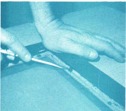
Step 2. Remove the old screen material by taking out the tacks or staples.
