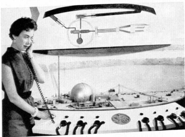
Model of 180,000 kilowatt power station to be constructed near Chicago, is given last-minute check before shipment to the United Nations conference at Geneva. A 200-foot sphere will house the atomic reactor and turbine-generator.
