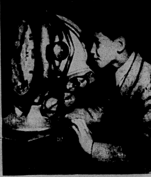
EASY STUDY —This oversized model of a watch, in the German Museum Physics department at Munich, affords a student an easy study of the workings without risk of breakage.
