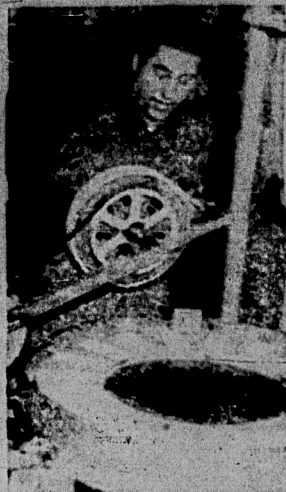
—Photo by Al Ternes Charles Burridge places an abrasive wheel on painted concrete strips. The wheel simulates the effect tires have on painted lines on highways. Purpose of the wearing action is to test the durability of various paints.
