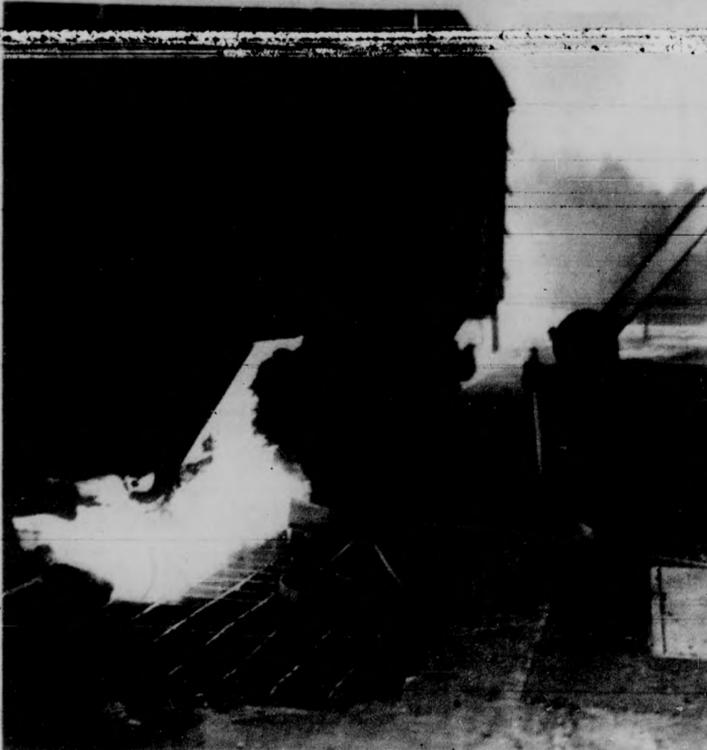
OVERSIZED BLOWTORCH--Gerry Williams sets a giant blowtorch under a coal-car at the South Power Plant. The torch melts the ice formed at the bottom of the hopper cars
