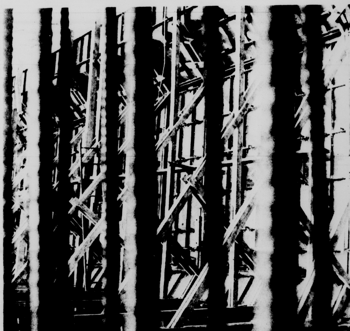
PATTERNS IN PROGRESS--Stands of reinforcing rods and wall forms present unusual picture possibilities at the new East Lansing sewage plant. The plant which is to be completed next summer will serve East Lansing, MSU and Meridian Township, replacing the overloaded plant near Brady Group.
