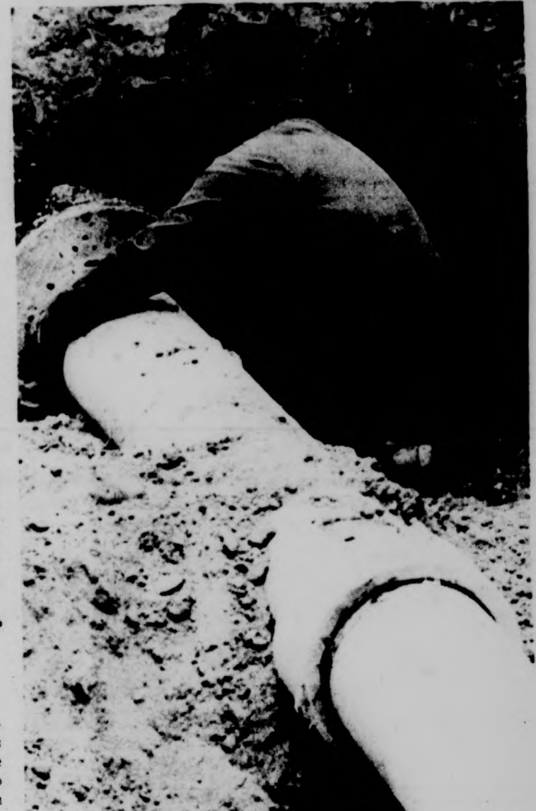
RUSTIC —Out with the old and in with the new seems to be a fitting comment on the replacement of an old pipe line that rusted out in the new athletic field. Workmen are shown putting in the new pipe line. Photo by Cal Crane
