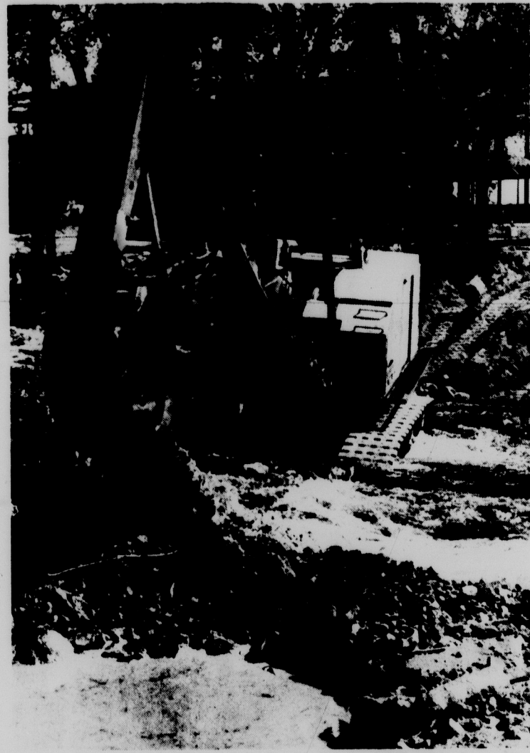
TO THE BOTTOM OF THE RED CEDAR--Steam shovel is being used to dig a channel for a pipe to be laid across the river between the railroad bridge and the bridge behind Computer Center.
