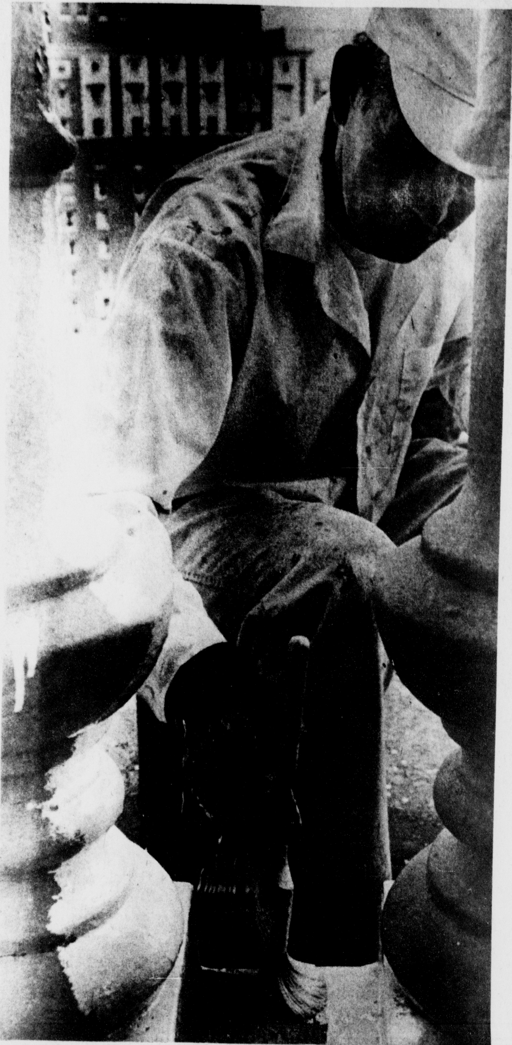
J.A. LaFontz spreads white epoxy onto the Capitol dome in Lansing, covering a yellow-green primer coat that was applied earlier.
