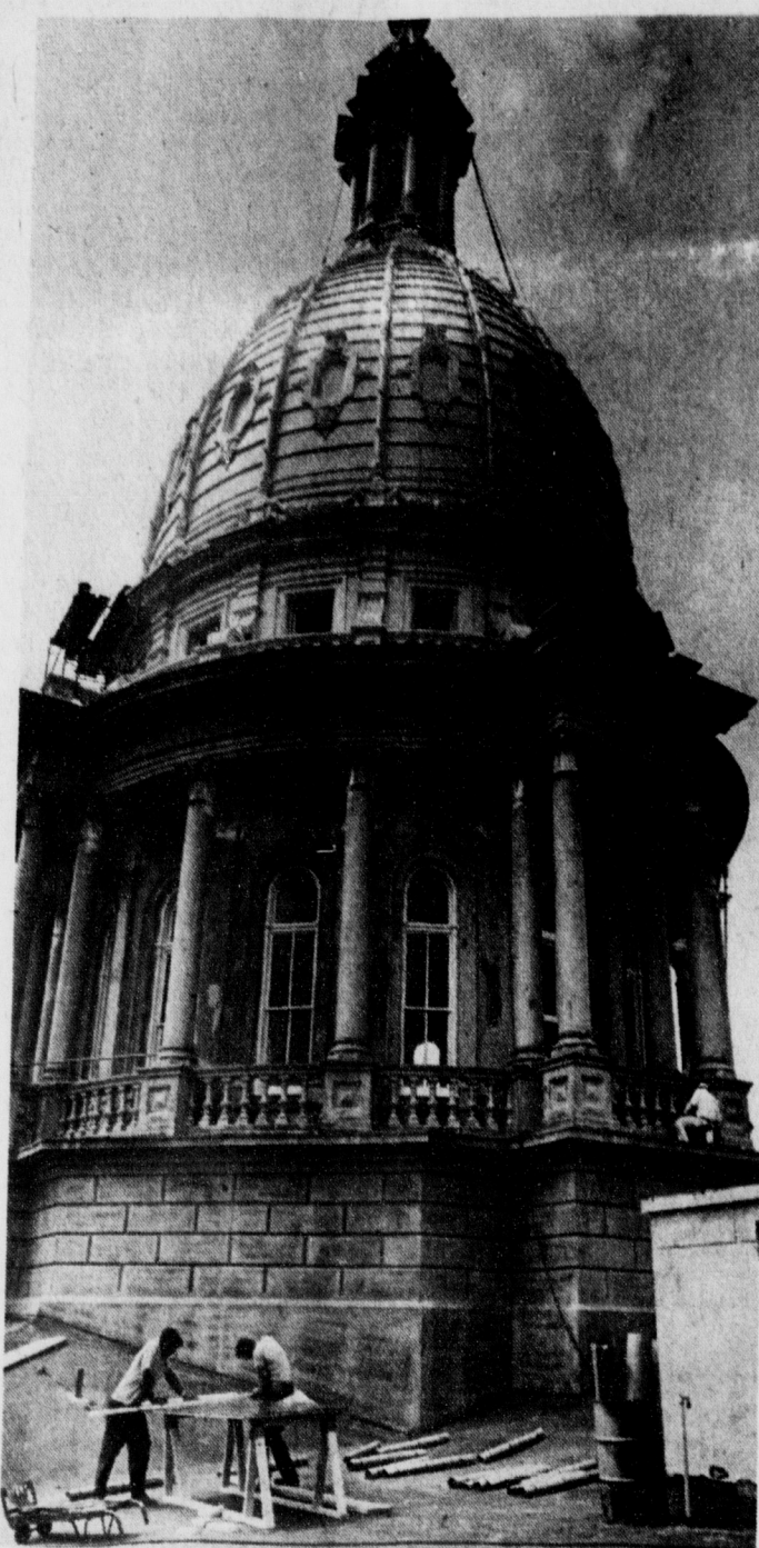
Michigan's Capitol dome looms above sheet-metal workers as they cut sheets of lead to be placed around the dome to prevent water damage.
