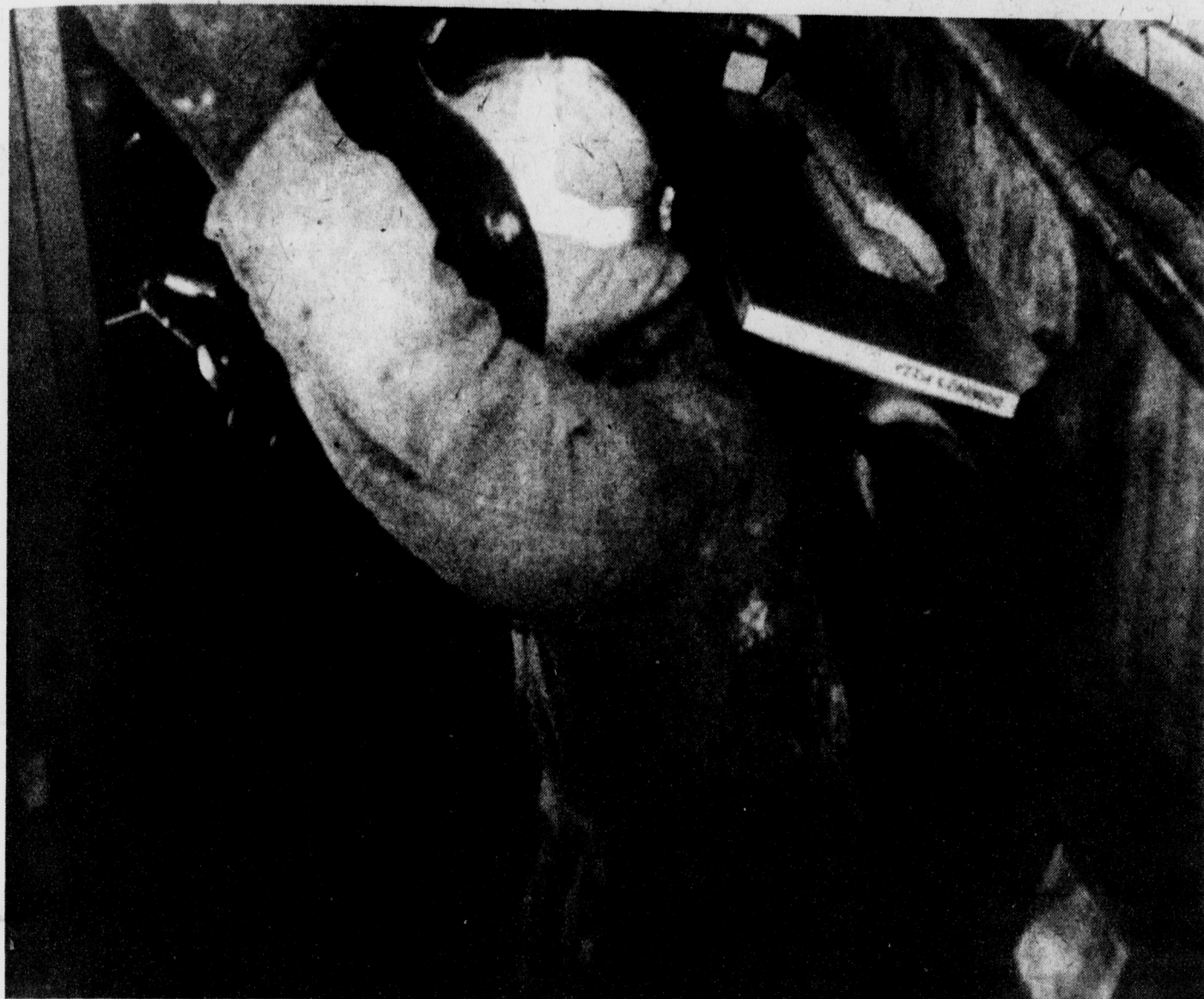
A student welder repairs a portion of the steam heating pipes that run under MSU's turf and concrete. The tunnels holding the pipes extend for five miles under campus.
