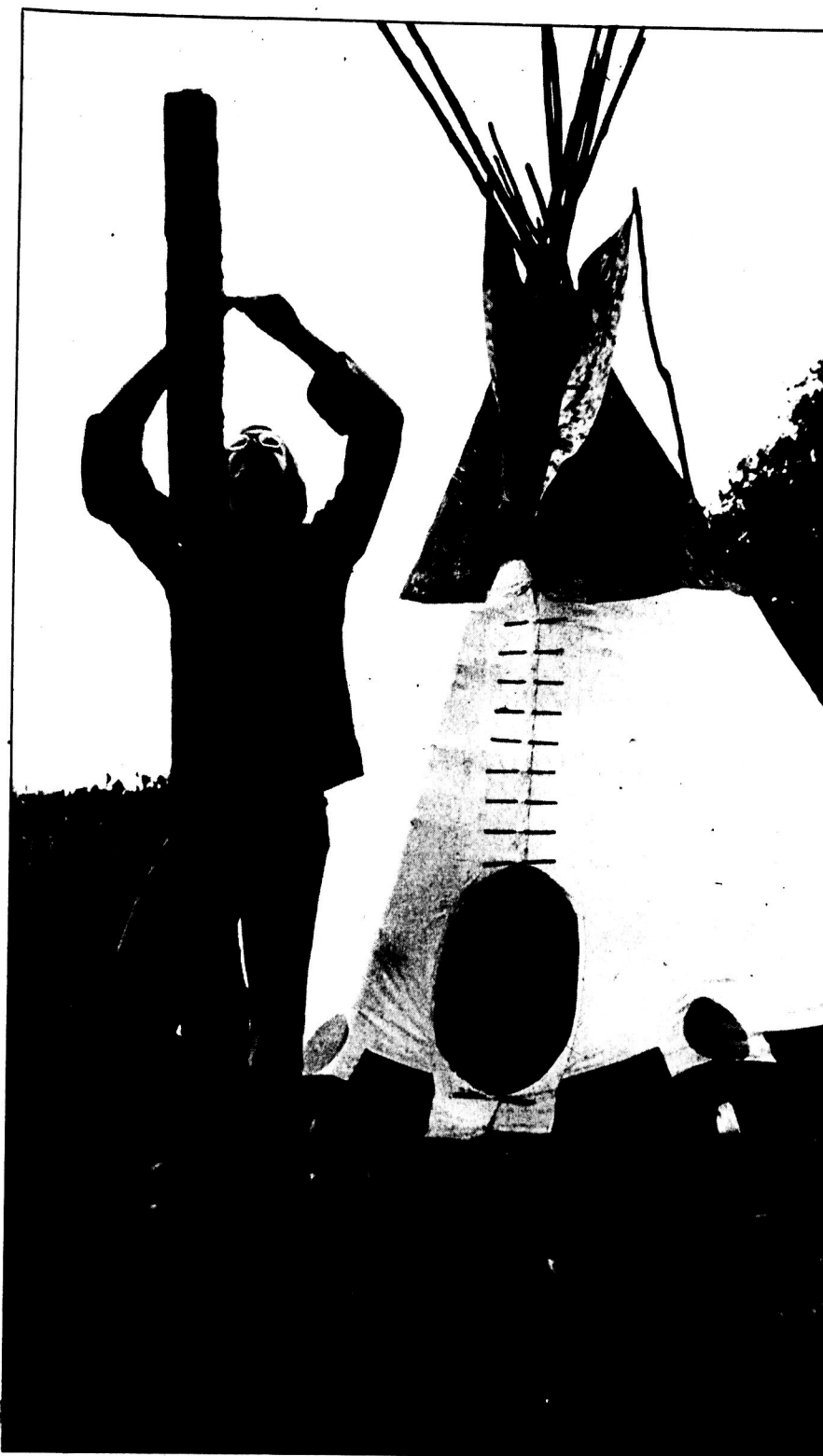
Pritchard adjusts the smoke flaps on his Sioux-style tepee. The flaps are designed to regulate the currents of air carrying smoke out through the chimney of the tipi.
