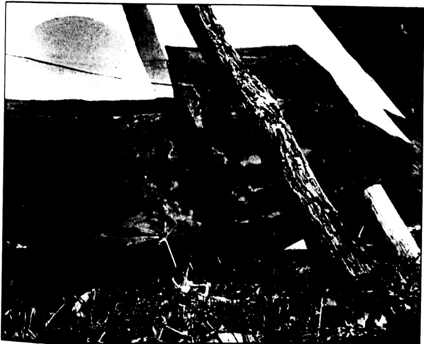
The exterior skin does not cover the entire tipi but leaves a gap of about 4 inches at the bottom. This allows air to flow in through the tipi and create drafts that eventually draw the smoke out the chimney while leaving the warm air in. The painted symbols are from patterns used by the Sioux.
