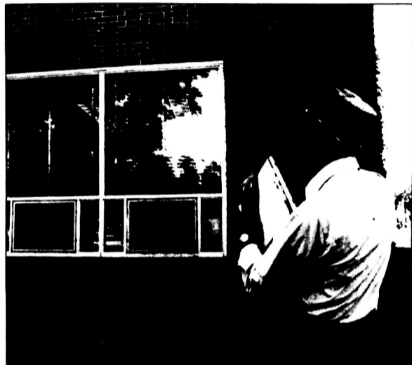
State News Deborah J. Born The exterior masonry of all MSU buildings is checked periodically by MSU Grounds Maintenance personnel. Ralph Wight looks for cracks in the Student Services Building that can cause structural, insulation or waterproof problems if left unattended.
