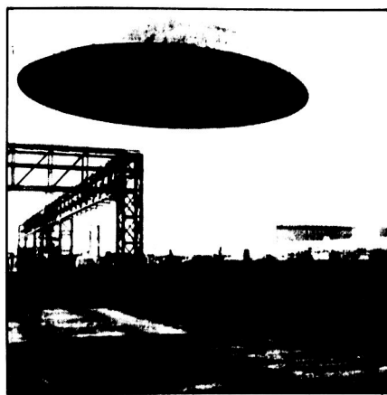
This is not an Unidentified Flying Object. It is a large styrofoam cover for a water treatment plant in Saginaw. The dome weighs 6,500 pounds, is 60 feet wide and 15 feet high. The treatment plant is expected to be in operation by next spring.
