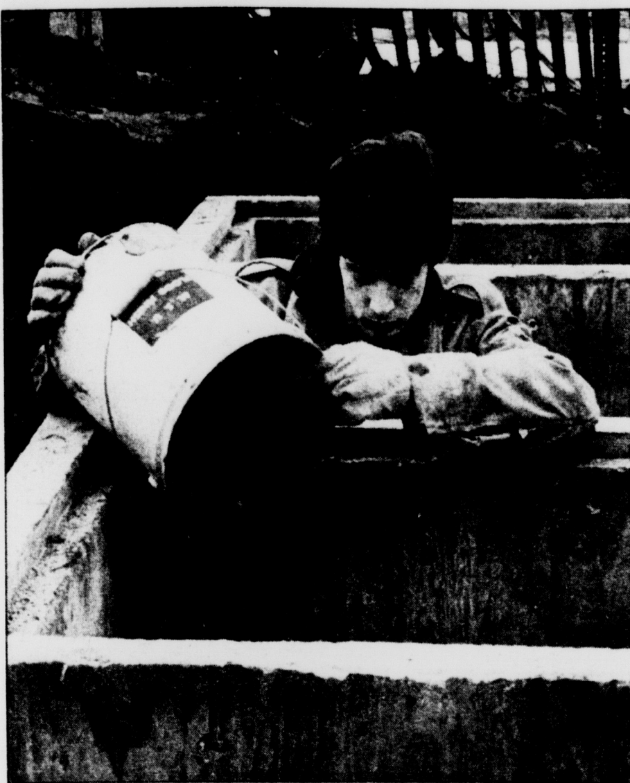
State News, Susan M. Pokrefsky Though it's not an episode from "Rocky," it is a pretty "rocky" episode! Physical Plant worker David Kemper pours rocks into the ventilation shaft in front of Wonders Hall. The rock-filled shaft allows a steam-carrying vault underneath to cool without letting rain water seep down.
