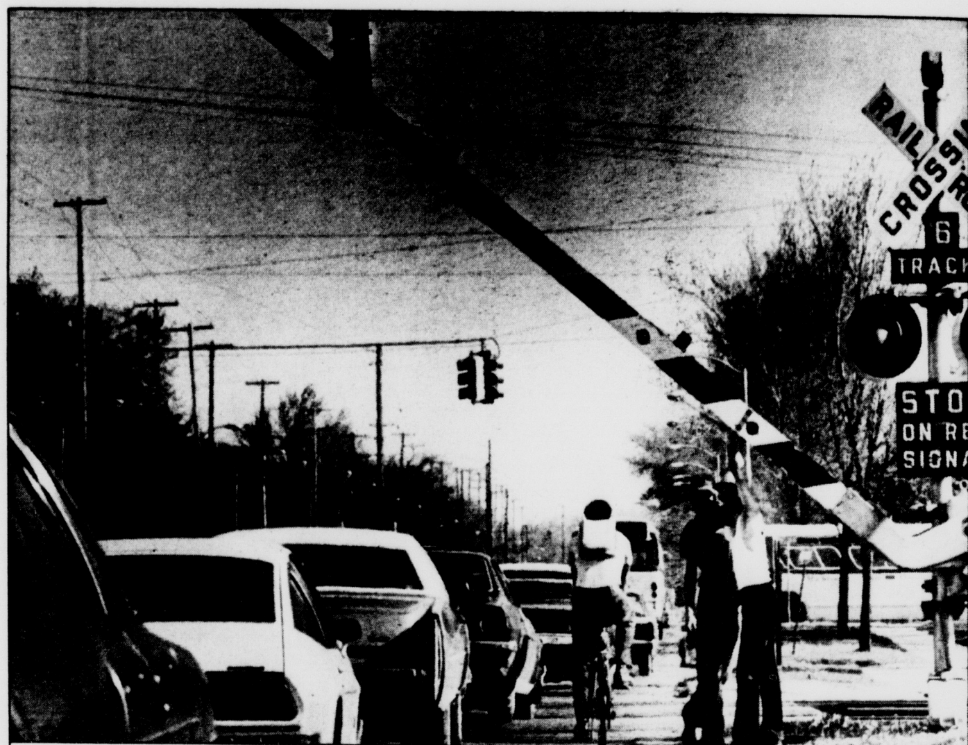
Did you ever get frustrated enough to get out of your car and lift the crossing gate that's causing a traffic jam during rush hour, when there's no train coming? Mike Dailey and Mark Link, who work for Grand Trunk & Western Railroad, felt that way. A malfunction in the track circuit was the cause.
